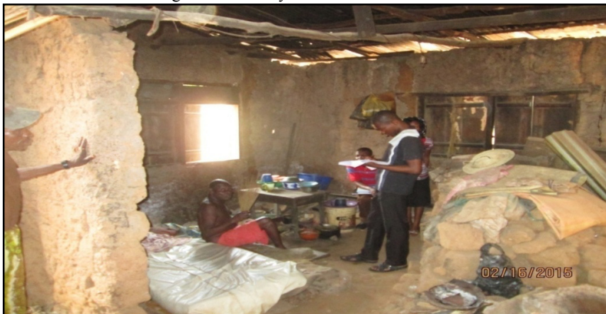
Plate 1: An inhabited house whose dilapidation was caused by flyrock and vibration at Lamulo village, located few meters from a quarry site in Oluyole LGA. Oyo State
