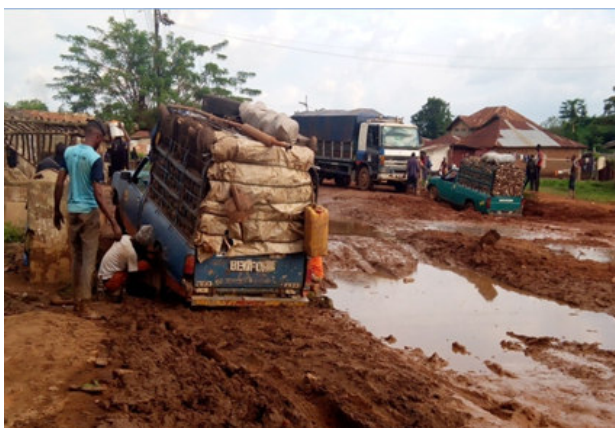
Plate 1: Bad road network at Ijaye in Oyo state, Nigeria; a challenge to transportation of farm produce, which could result in post harvest losses.
